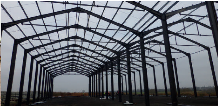
Industrial Grain Store - under construction
