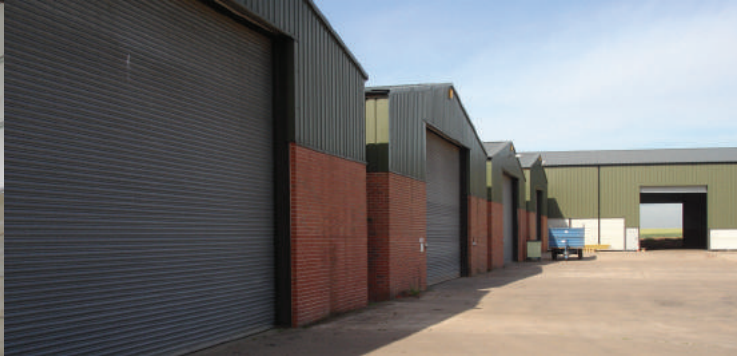
A range of industrial structures each 18m Span x 60m Long x 6m to Eaves
