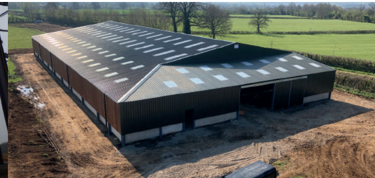
Riding School being 20m wide x 48m long x 5m to eaves.
